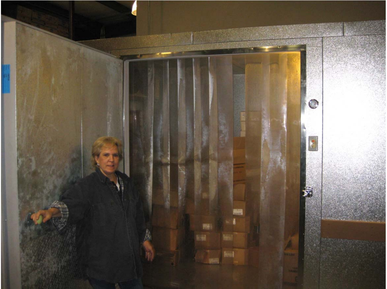
Figure 3: New Walk-In Freezer at North Kent Service Center
