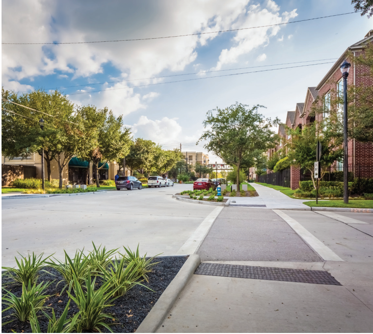
Bagby Street with Bulb-out Curb (Image: Midtown Houston)
